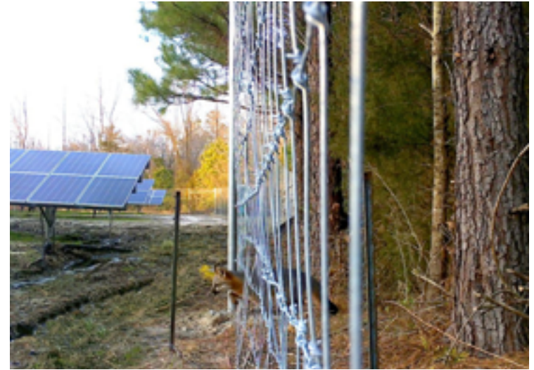
Figure 6-2. Wildlife-friendly fencing at a solar facility in Moore County, North Carolina (Credit: Liz Kalies, The Nature Conservancy)
