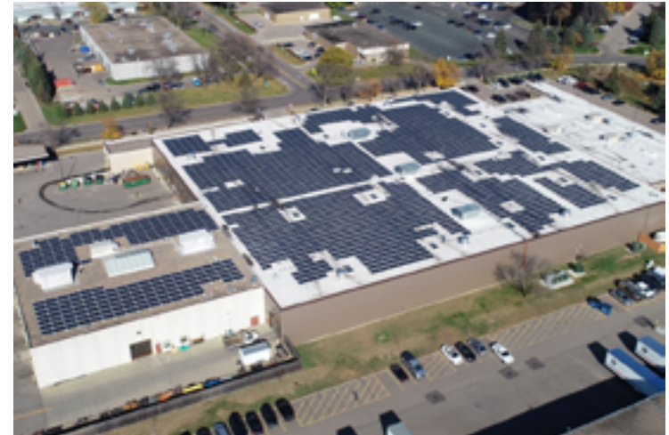
Figure 7-3. A 618 kW shared solar project in Edina, Minnesota, for which the city serves as a backstop subscriber (Credit: Impact Power Solutions)
