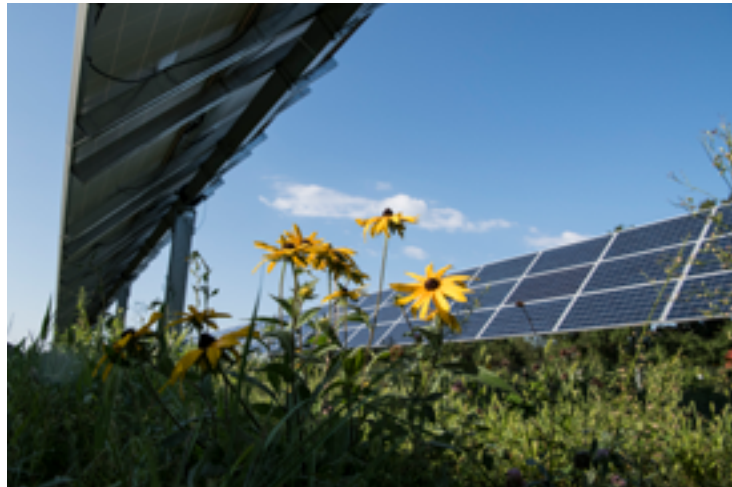
Figure 5-2. Pollinator-friendly ground cover at the Aurora Solar Project in Chisago, Minnesota (Photo by Dennis Schroeder, NREL 53020)
