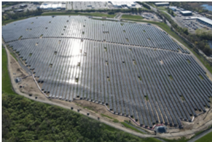
Figure 5-1. A 25 MW solar facility on the former Combe Fill North Landfill Superfund site in Mount Olive Township, New Jersey (Credit: CEP Renewables)
