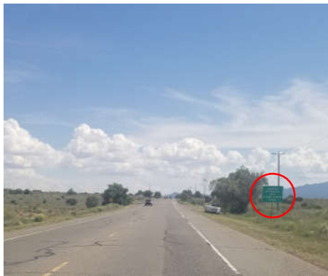
Figure 8: NM 14 Southbound Speed Guide Sign
